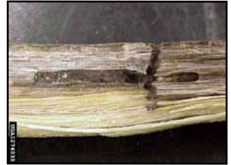
Figure 3. Empty gallery following Cnestus mutilatus damage.
